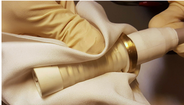
Figure 10 - Cleaning the cable connector
